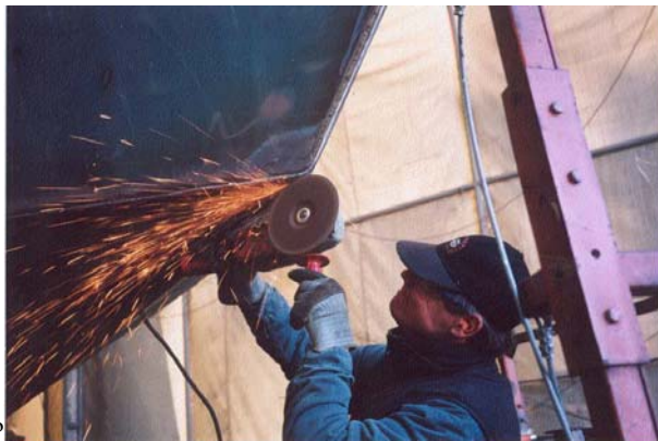
Figure 2. Manual Weld-bead grinding in medium sized structures
