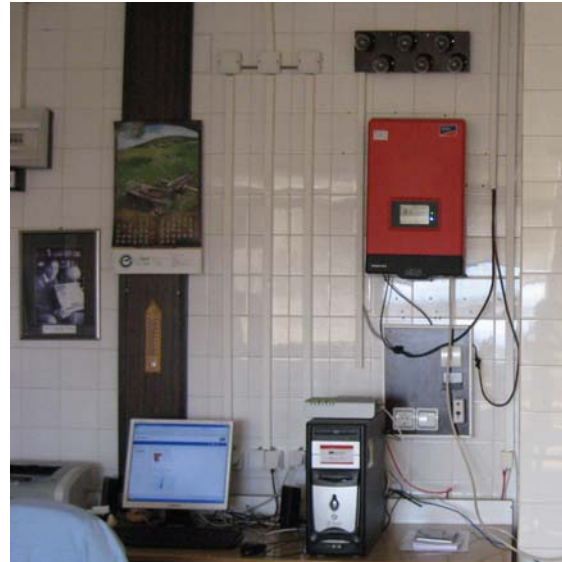
Figure 7. Part of the interior of Solar Energy Laboratory with inverter and SUNNY WEBBOX
