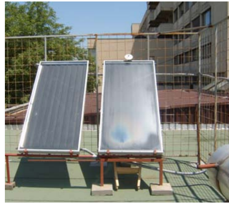
Figure 21. Flat collectors on the roof of Civil Engineering faculty in Niš
