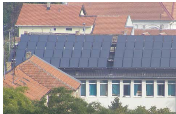
Figure 4. Solar collectors on the roof of Youth home Angelina Kojić Gina in Zrenjanin
