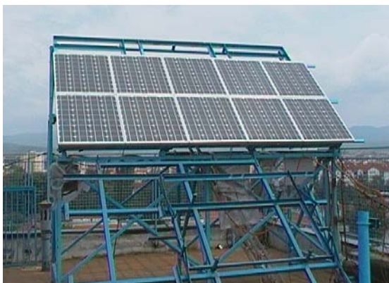
Figure 16. PV solar plant of 600 W with monocrystalline silicon solar modules on the roof of the Faculty of Science and Mathematics in Niš
