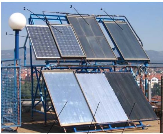
Figure 15. Part of Laboratory for solar energy on the roof of the Faculty of Science and Mathematics in Niš: 1) solar module, 2) hybrid collector with solar cells made of monocrystalline silicon, 3) hybrid collector with solar cells made of amorphous silicon, 4) flat collector with spectrally selective absorber, 5) flat collector with non-coloured absorber, 6) non-coloured absorber, 7) spectrally selective absorber
