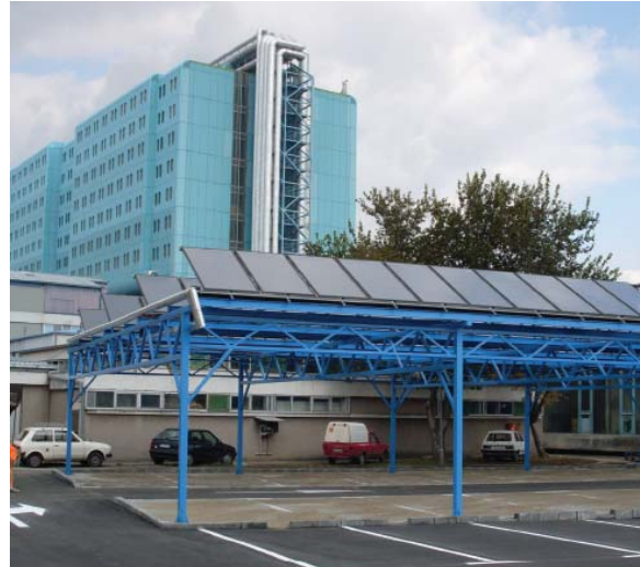
Figure 3. Solar collectors in Zrenjanin's hospital Dr Đorđe Jovanović
