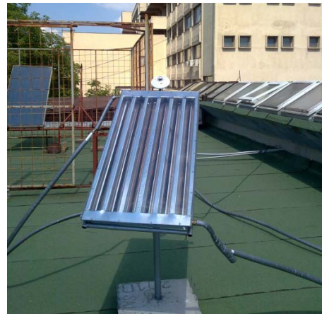
Figure 22. Compound Parabolic Collector- CPC-2V for middle temperature conversion of sun radiation into thermal on the roof of the Faculty of Civil Engineering in Niš
